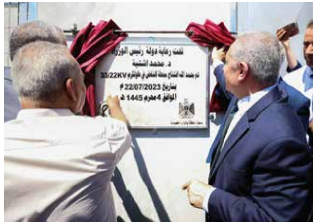
Prime Minister Dr. Mohammad Shtayeh inaugurates Tulkarem low-voltage plant for addressing the electricity crisis in the governorate.
